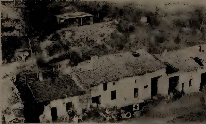
1. Dressing station post at Dommartin, buildings on the side of the hill have enormous bomb-proof Dug-outs back of them built by the Germans.
